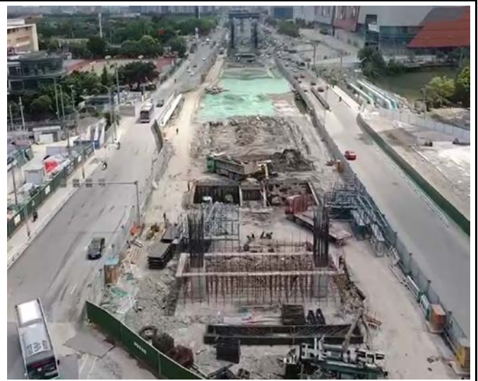
2 标桩基承台施工 (2021. 03)
