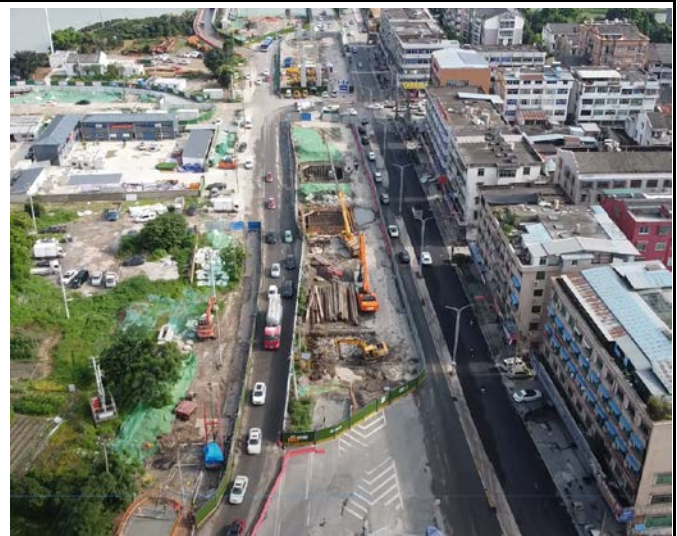
3 标桩基承台施工 (2021. 03)
